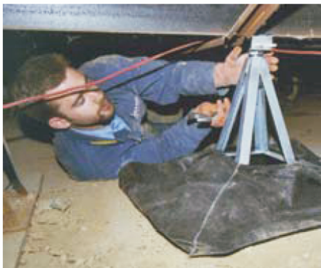
Technician completes bolting the Sure Safe steel buttress to the steel chassis beam under a HUD-Code home. Note how the base of the galvanized steel buttress is enclosed by the patented geotextile form bag.
