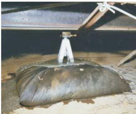
The concrete fills the bag forming a solid concrete attachment measuring approximately 6-1/4 sq. ft. At the right one of the temporary support jacks is seen which is utilized to level and hold the home firmly until the concrete hardens in the permanent buttress system members.
